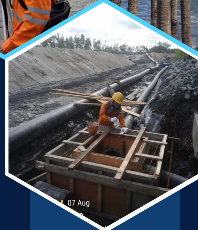
Rebar & Formwork Fabrication
