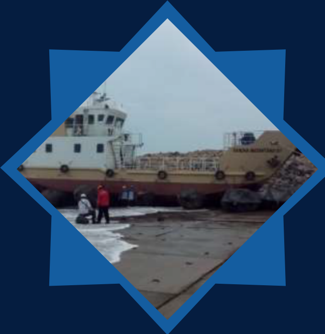
JETTY FOR LSF COMPLETED
