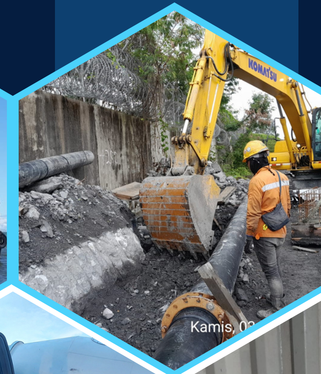
Excavation and Grading
